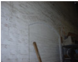
Segmental arched opening in south wall
