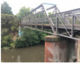
Walmer Street Bridge - view from south bank - 2019
