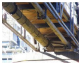
Walmer Street Bridge - pipe from Dights Falls Scheme suspended under bridge - 2019
