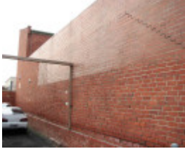
52 Edward Street Bendigo wall
