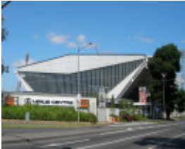
OLYMPIC SWIMMING STADIUM SOHE 2008
