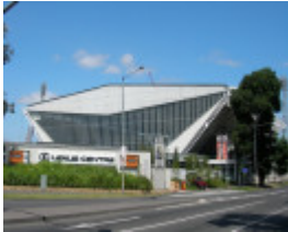
OLYMPIC SWIMMING STADIUM SOHE 2008
