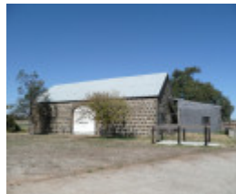
JUNCTION LODGE SOHE 2008
