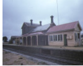
1 carlsruhe railway station trackside view sep1984
