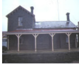
carlsruhe railway station platform view sep1984
