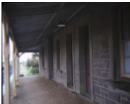
carlsruhe railway station verandah sep1984
