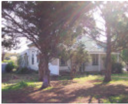
Federation period weatherboard residence
