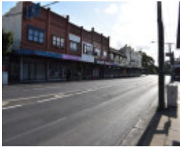
94-112 Bell Street, Coburg
