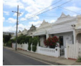
View along terrace row
