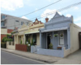
View along terrace row
