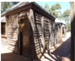
Rear of Post Office
