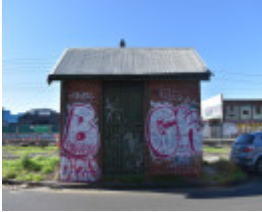
Colebrook Street substation
