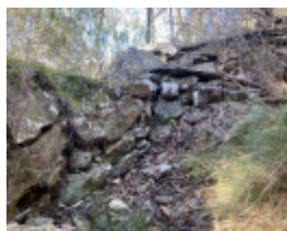
main trench overlooking road
