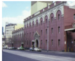
carlton brewery external front swanston street
