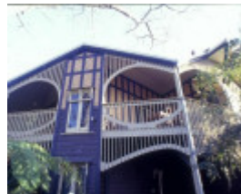
chadwick house the eyrie eaglemont south east verandah detail she project 2003
