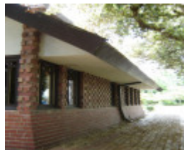
H2091 Lippincott House Glenard Dr Heidelberg Side Elevation Nov2005 mz
