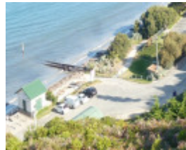
Pier boat ramp from above
