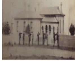
First cable station and PO
