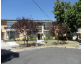
Ardene Court Flats, 11 Ardene Court, Hawthorn
