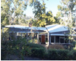
'Milston House', 6 Reeves Court KEW
