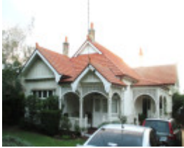
Merledon, 16 Beaconsfield Road, Hawthorn East
