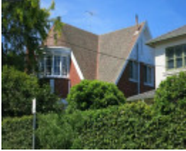
Mombah, 9 Widford Street Hawthorn East
