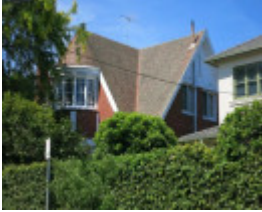
Mombah, 9 Widford Street Hawthorn East
