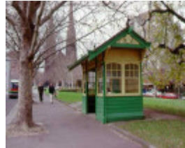
1 tram shelter cnr macarthur st & st andrews pl east melbourne
