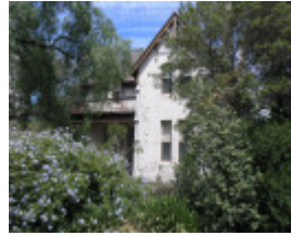
HOLY TRINITY CHURCH, VICARAGE AND HALL SOHE 2008
