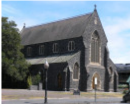
Holy Trinity Church, Vicarage and Hall SOHE 2008
