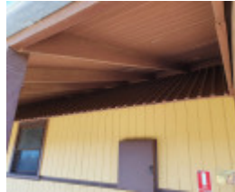
2022, Type A ventilated roof on the Former Irymple Railway Station building showing the batted timber inner roof and ventilator
