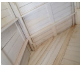
2020, interior of roof
