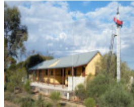
2022, Former Irymple Railway Station Building, platform side (signal not from Irymple)
