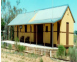
August 2022 Former Irymple Railway Station Building
