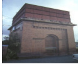
Elmore Railway Station Water Tower (1984)
