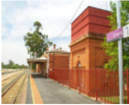
Elmore Railway Station and Water Tower
