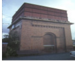
Elmore Railway Station Water Tower (1984)
