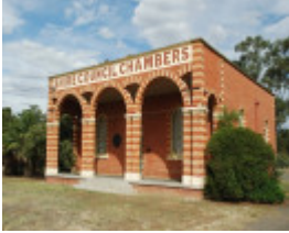
Former Huntly Shire Council Chambers
