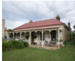
FORMER ST ANDREWS PRESBYTERIAN CHURCH AND MANSE SOHE 2008
