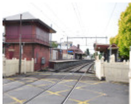
View north from the Anderson Street Railway Crossing shows main structures of the complex
