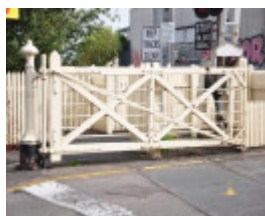
Interlocking Railway Crossing Gate (2023)
