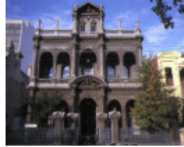
1 Benvuta Drummond Street Carlton front view
