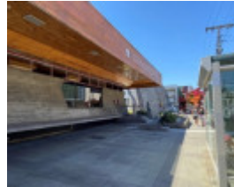
2025 St Kilda Public Library viewed from Carlisle Street
