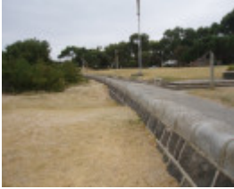
21305 Bluestone retaining wall
