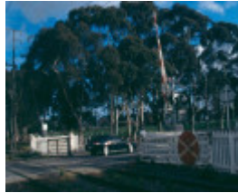
Brunswick Road Level Crossing Gates
