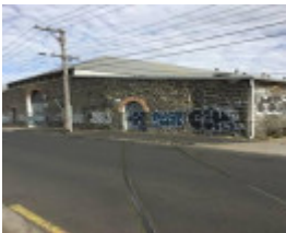
Industrial sidings Colebrook Street.jpg
