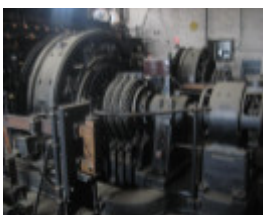
Substation - Rotary converters
