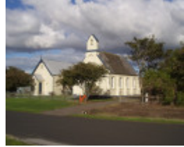
Church & Hall, Church Road Bellarine - Photo 1
