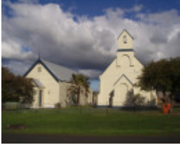
Church & Hall, Church Road Bellarine - Photo 1
