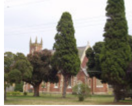
St James Anglican Church, Drysdale - Exterior Side View - 2
