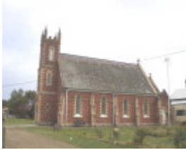
St James Anglican Church, Drysdale - Exterior Side View
