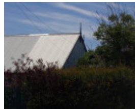
27 Harding Street, Portarlington - Exterior - Roof
