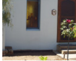
27 Harding Street, Portarlington - Exterior Front Door
