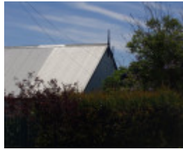
27 Harding Street, Portarlinton - Exterior - Roof
