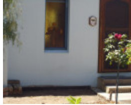
27 Harding Street, Portarlinton - Exterior Front Door
