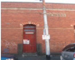
Brunswick cable tram engine house substation entrance
