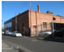
Brunswick cable tram engine house - substation
