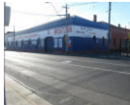
Brunswick cable tram engine house
