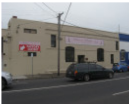
Brunswick cable tram engine house 261-63 Brunswick Road
