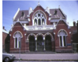
1 carlton court house drummond street carlton front elevation feb1985
