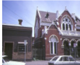
carlton court house drummond street carlton front corner elevation feb1985
