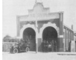
Geelong West Fire Station c.1922_resize.jpg
