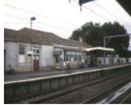
1 werribee railway station comben street werribee rear elevation oct1996
