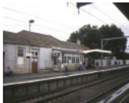
1 werribee railway station comben street werribee rear elevation oct1996
