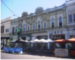
'Salisbury Buildings', Hobsons Bay Heritage Study 2006
