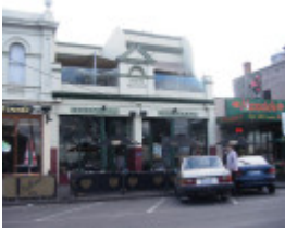
Modern Building at 213- 215 Nelson Place WILLIAMSTOWN, Hobsons Bay Heritage Study 2006
