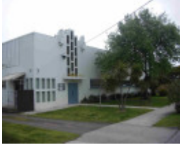
Red Robin Hosiery Factory (former), Hobsons Bay Heritage Study 2006
