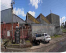
McKenzie and Holland Factory Complex (former), Hobsons Bay Heritage Study 2006
