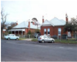
Police Station, Sergeant and Watch house Keeper Quarters (former), Hobsons Bay Heritage Study 2006
