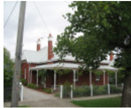
Police Station, Sergeant and Watch house Keeper Quarters (former), Hobsons Bay Heritage Study 2006 - No. 10
