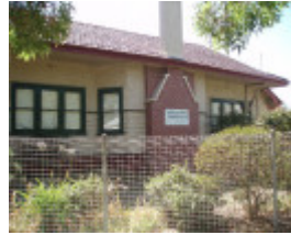
Williamstown Croquet Club Pavilion, Hobsons Bay Heritage Study 2006
