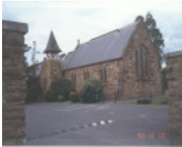
22376 Holy Trinity Anglican Church - 792-800 Church Street, Doncaster (1)
