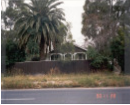
22397 House - 50 George Street, Doncaster
