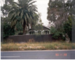
22397 House - 50 George Street, Doncaster
