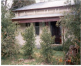
22398 House - 88-90 George Street, Doncaster
