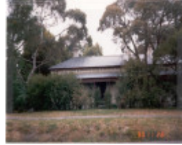
22398 House - 88-90 George Street, Doncaster (2)
