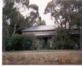
22398 House - 88-90 George Street, Doncaster (2)
