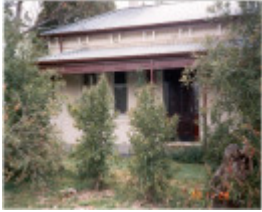
22398 House - 88-90 George Street, Doncaster
