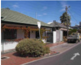
Cox's Garden Heritage Precinct, Hobsons Bay Heritage Study 2006
