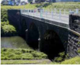
Melbourne-Geelong Road Precinct BROOKLYN, Hobsons Bay Heritage Study 2006
